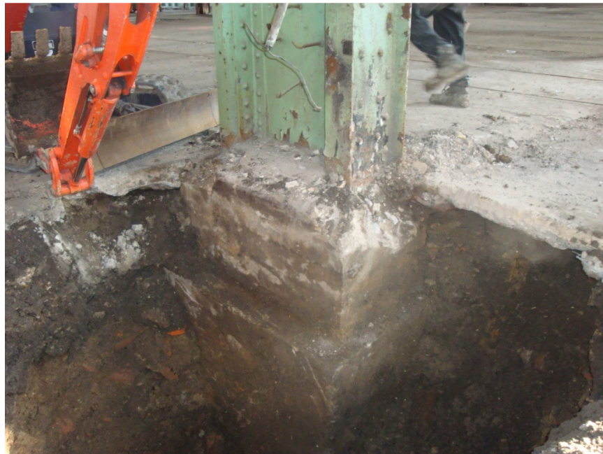
Photo #5: Concrete pier in test pit location
