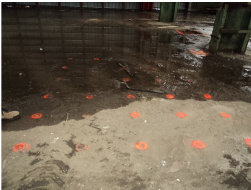
Photo #41: Typical slab-on-grade embedded anchors
