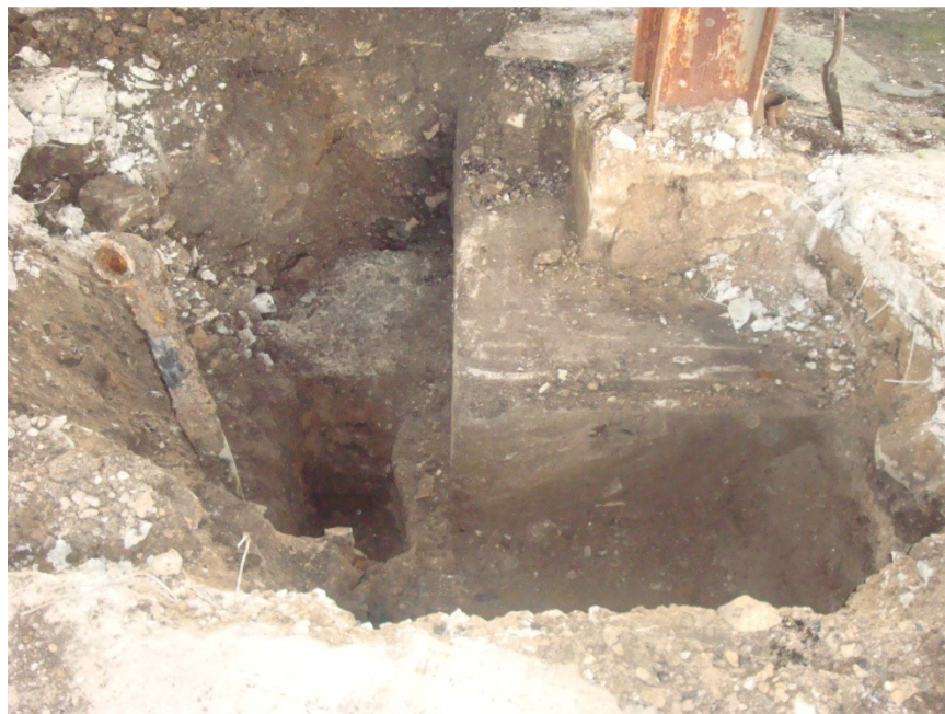
Photo #35: Test Pit #1 - Face of potential Grade Beam
