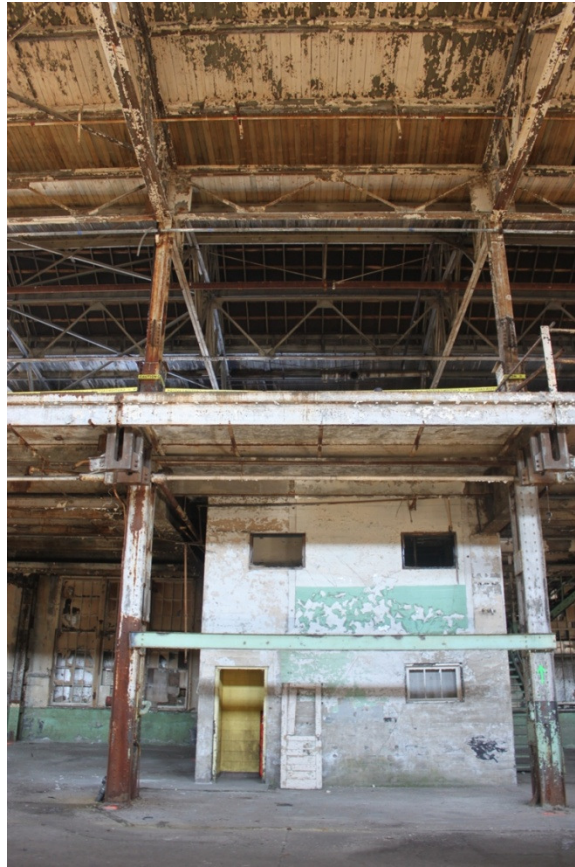
Photo #4: Lateral stabilizing elements of mezzanine bay (slab and shaft)
