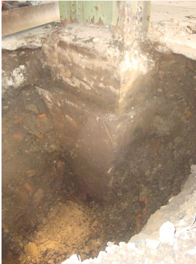
Photo #36: Test Pit #2 - Footing / Caisson Cap
