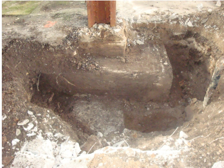
Photo #34: Test Pit #1 - Footing / Caisson Cap
